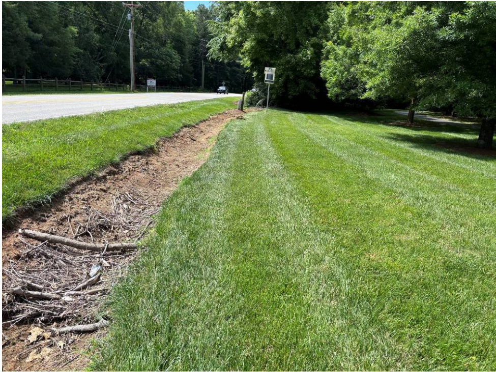
Photo 19: Looking south from the access road at the existing ditch.
