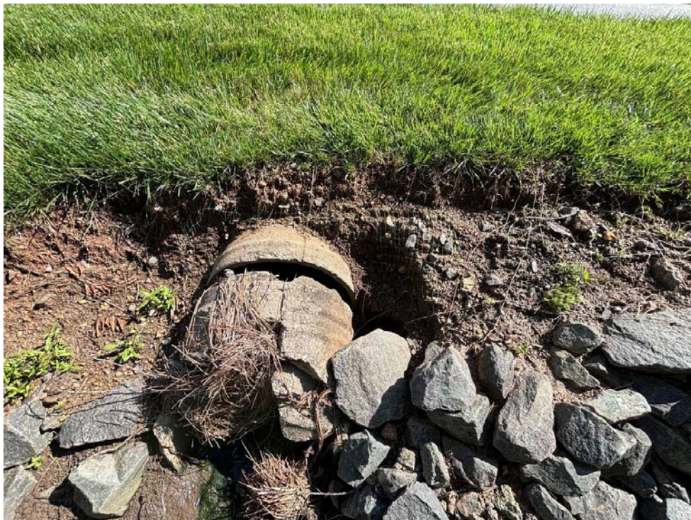
Photo 20: Upstream end of the RCP culvert under Joe Kerr Road.
