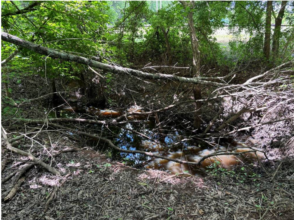
Photo 7: Deep ponded area of water on the west side of the trail. School fence is in the background.
