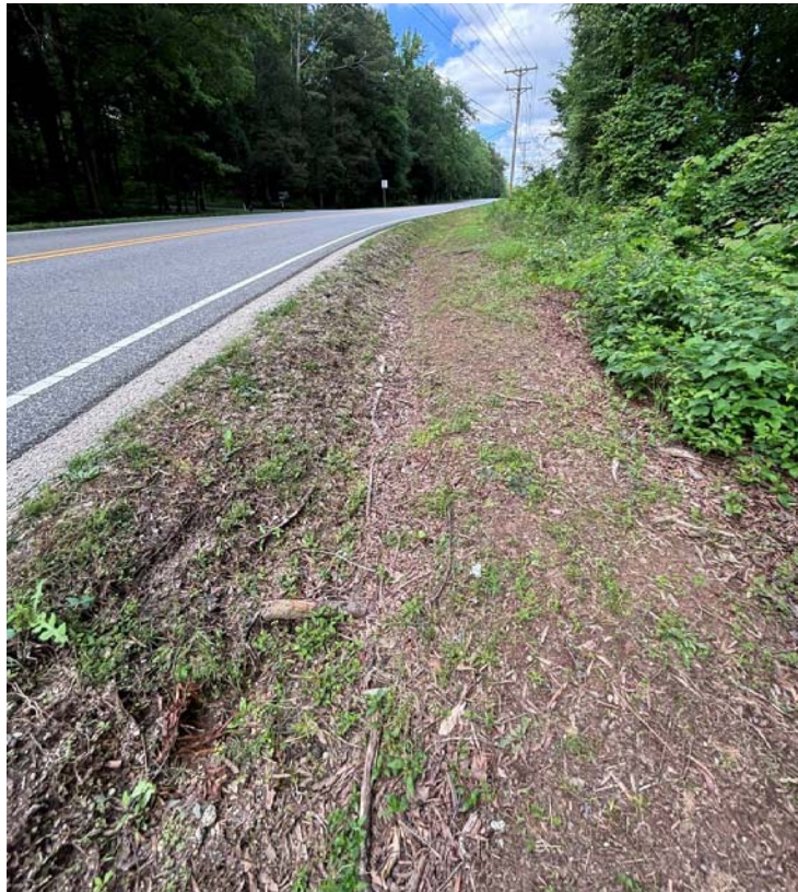
Photo 21: Existing ditch along the wood line, looking south.
