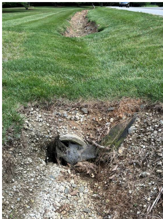
Photo 16: RCP culvert under the access road, looking north.
