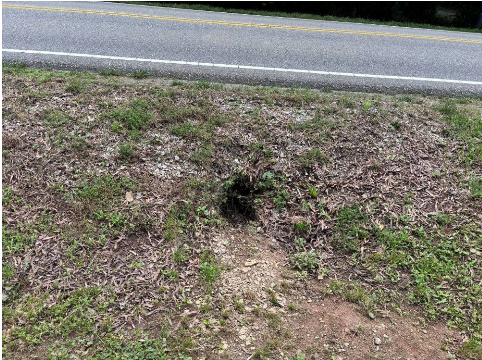
Photo 3: Outfall of culvert under Marvin School Road
