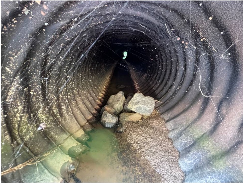
Photo 19: Upstream end of the CMP under Joe Kerr Road
