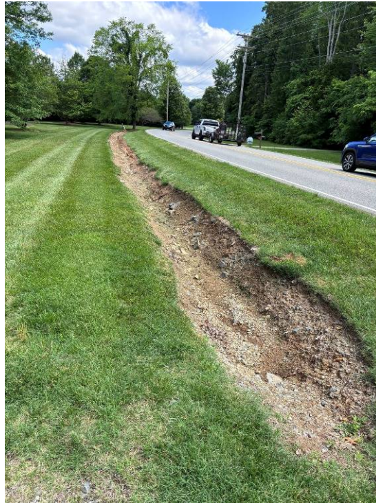
Photo 17: Roadside ditch downstream of the culvert and access road
