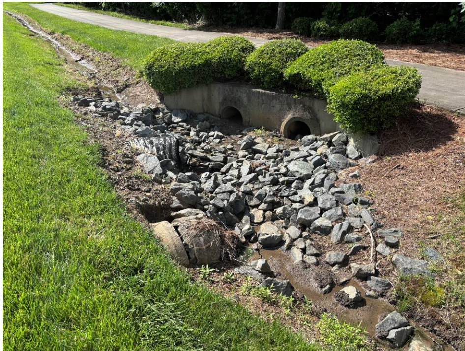
Photo 15: Headwall and RCP culverts under the trail.
