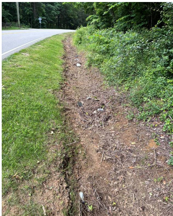
Photo 20: Existing ditch at wood line, looking south.
