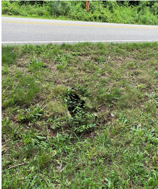
Photo 5: Upstream end of culvert on east side of Marvin School Road
