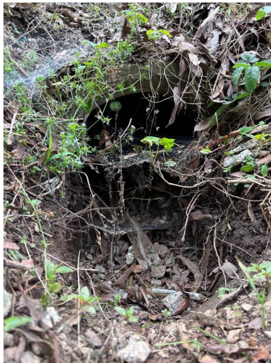
Photo 4: Close up of culvert outfall
