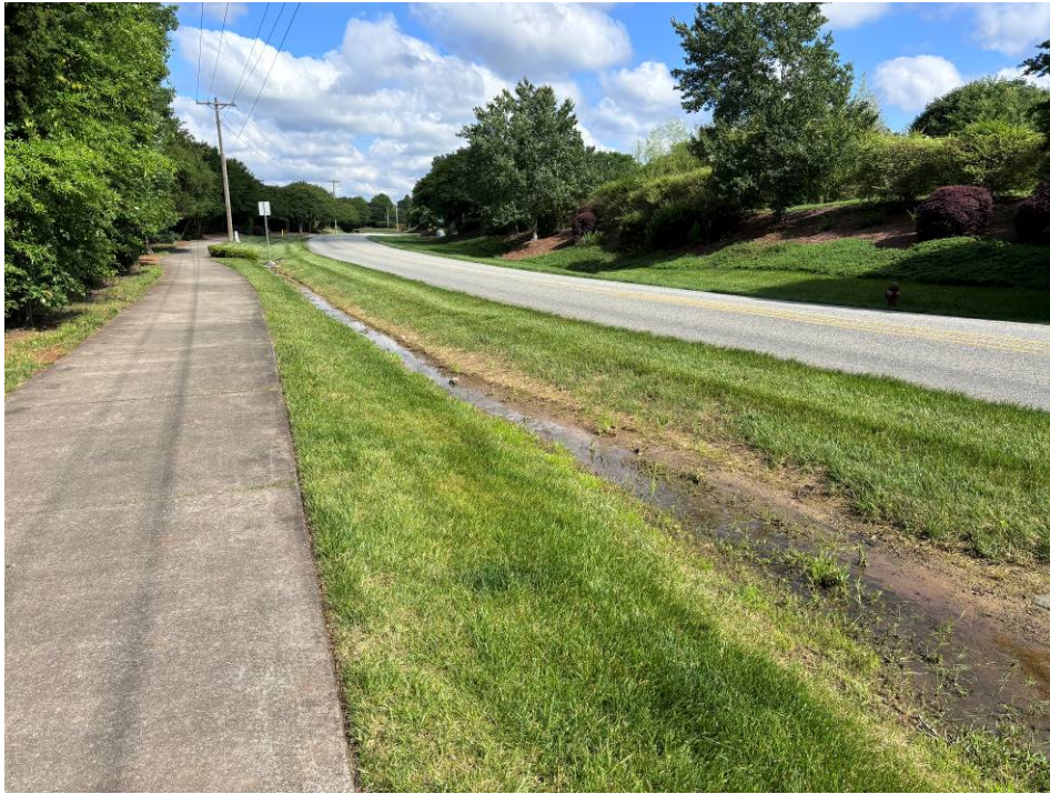
Photo 11: Shallow wet roadside ditch west of the woods.
