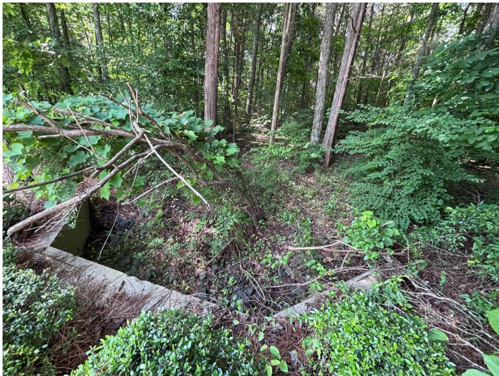
Photo 18: Headwall and upstream end of the culverts under the trail
