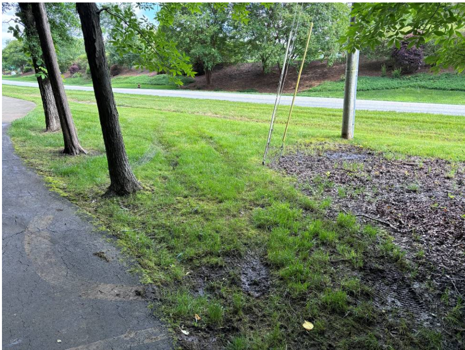
Photo 10: Trail heading west. Sediment and wet soils between the trail and road.
