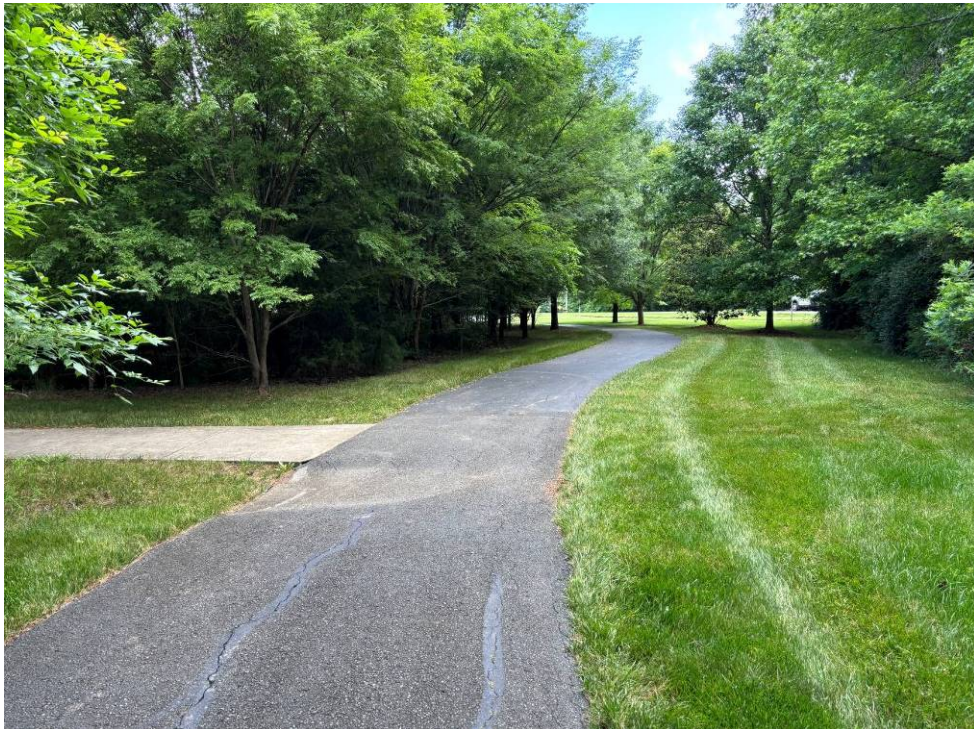
Photo 14: Connecting trail to Arborvitae Court. Note discoloration on the trail where water ponds.
