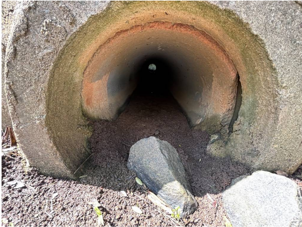
Photo 17: Downstream end of the RCP culvert under the trail.
